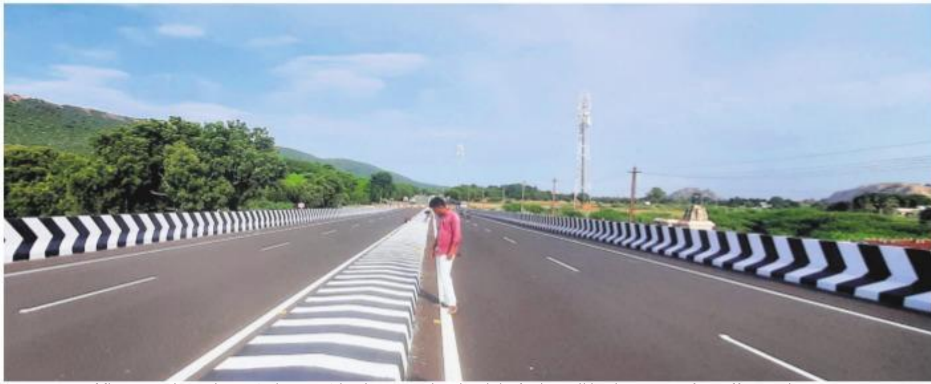
Construction of flyover on the Madurai - Cochin NH 49 has been completed and the facility will be thrown open for traffic soon | EXPRESS
